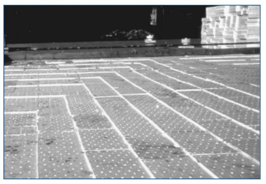
Stair-stepped EPS to create slope-to-drain.
